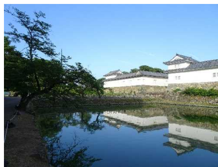
Photo 06 Second moat, stone walls, and ramparts
